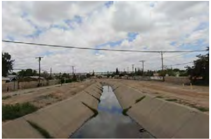
Canal that can serve as hike and bike trail. Trail infrastructure along irrigation canals should be planned and constructed in partnership with the irrigation district. Irrigation canals are required to be lined with concrete when any trail infrastructure is built along them.
