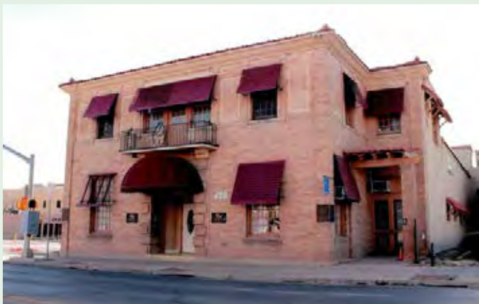
Exterior shot of the building before renovations.
