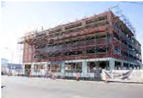
Building on Texas Avenue being repurposed into Class A office space.
