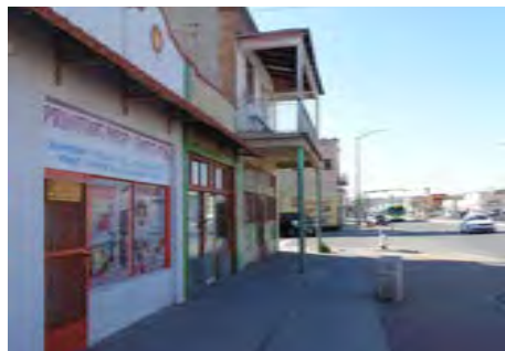
Traditional and local architectural styles dominate in this area, such as the two-story gallery shown here. While the building frontages are that of a pedestrian friendly main street, the design of Alameda itself encourages high speed travel and is difficult to cross.
