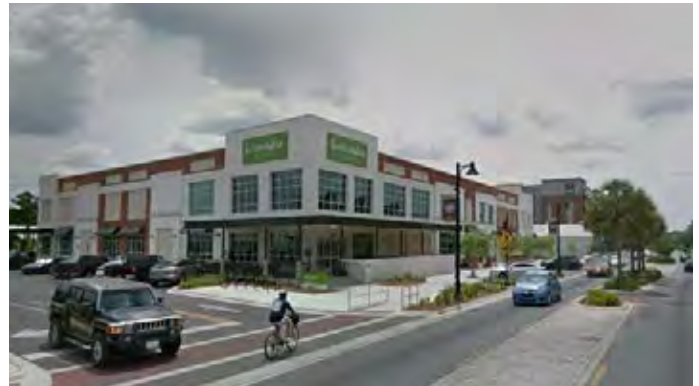
This national chain supermarket is fronted along the street instead of the parking lot and incorporates elements of street-oriented architecture (Tallahassee, FL).
