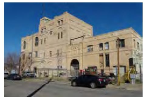
Industrial uses and warehouses, with an emphasis on produce, are located along the railroad. Some of the buildings have unique designs and are good candidates for adaptive reuse. The area’s produce markets and access to a variety of food products provides an economic base to build upon.
