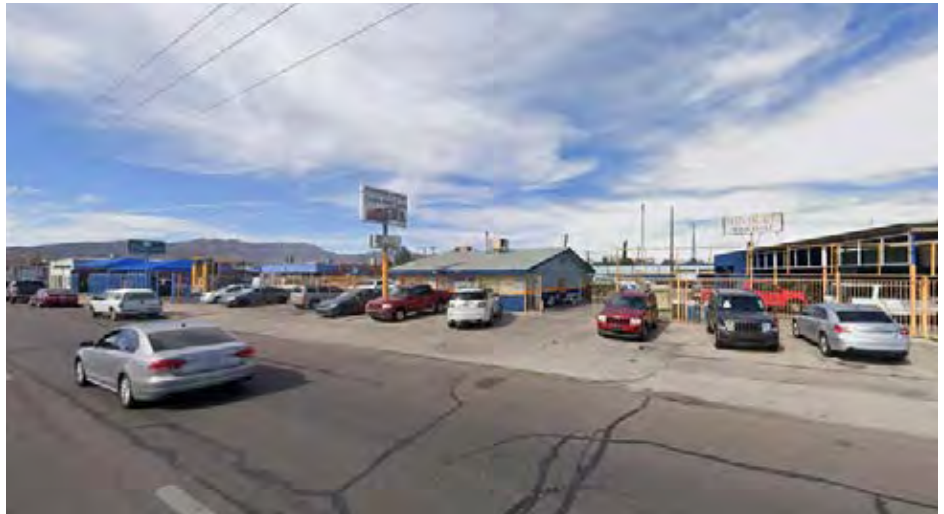
Existing conditions along longer stretches of Alameda Avenue
