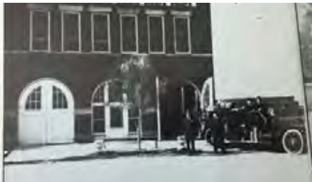
The East El Paso Fire Station (No.5), also known as the 1924 Democratic Primary Polling Place, was built in 1908 and still stands at Alameda & Texas Ave. It remains the oldest unaltered station in El Paso, Texas.
