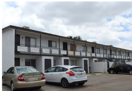
Multifamily Apartments along segment 5 of the Alameda corridor.
