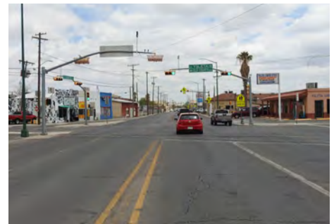
Most of Alameda Avenue consists of four travel lanes and either a center median with turn lane or a center two-way left-turn lane.
