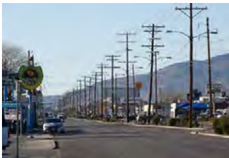
Relatively low traffic volumes and long open stretches of highway invite speeding, a concern to both area businesses and residents.
