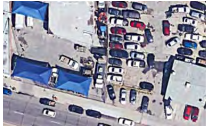
Existing conditions along longer stretches of Alameda Avenue
