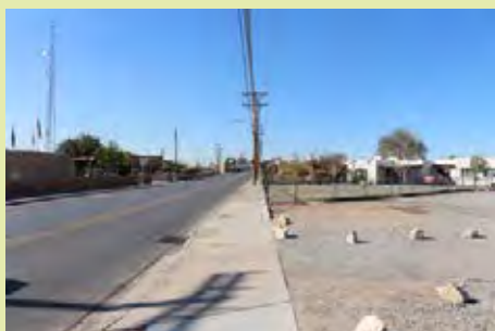
Socorro Road Existing Streetscape at Southside Road
