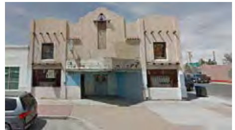
The Alameda Theatre, also known as The Mission Theatre, was built in 1940, which originally opened on March 15, 1941. As of today, the building stands vacant.
