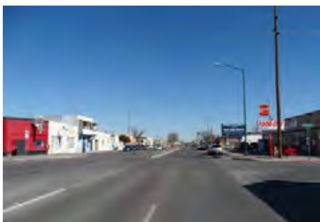
Alameda Avenue consists of four travels lanes with a center left turn lane and median in this segment. On-street parking serves the businesses as many parcels are too small to accommodate on-site parking. However, the street has highway features with wide lanes, minimal street trees and tall lighting. The street design does not match or support the land use and buildings alongside it.
