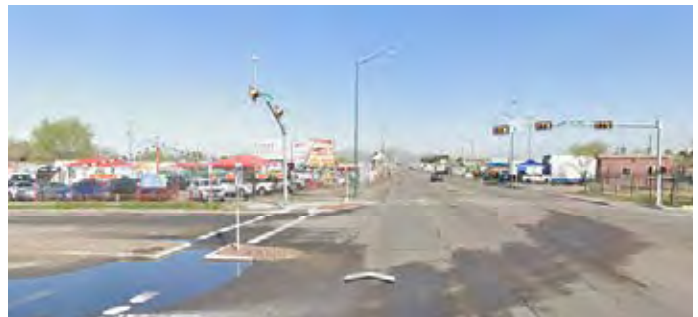
Example of typical flooding conditions along Alameda Ave hindering walking and transit use
