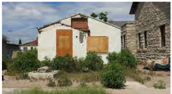
This vacant and boarded up house on Tobin Place near various other vacant infill parcels.
