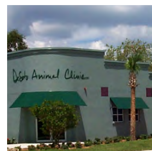
Awnings provide shelter at entrances and shade windows.
