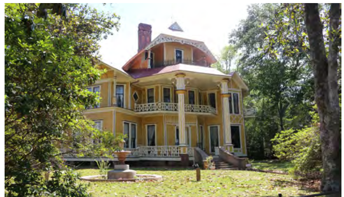
The historic Lapham-Patterson House has porches and large overhangs responding to the local climate.
