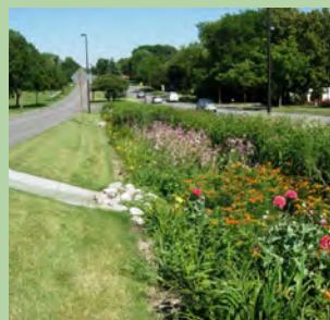
T2-T3: Bioretention swale
