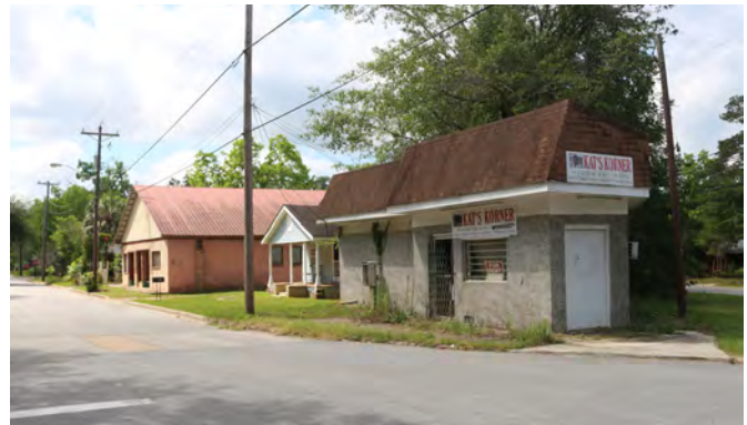
Vacant commercial properties in neighborhood centers
