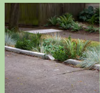
T3-T6: Planting strip trench
