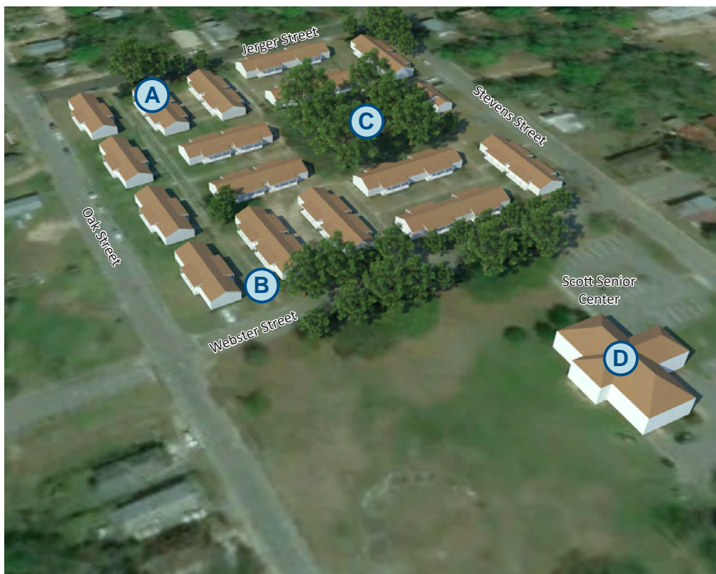
Faircloth Homes: Existing Conditions Aerial
