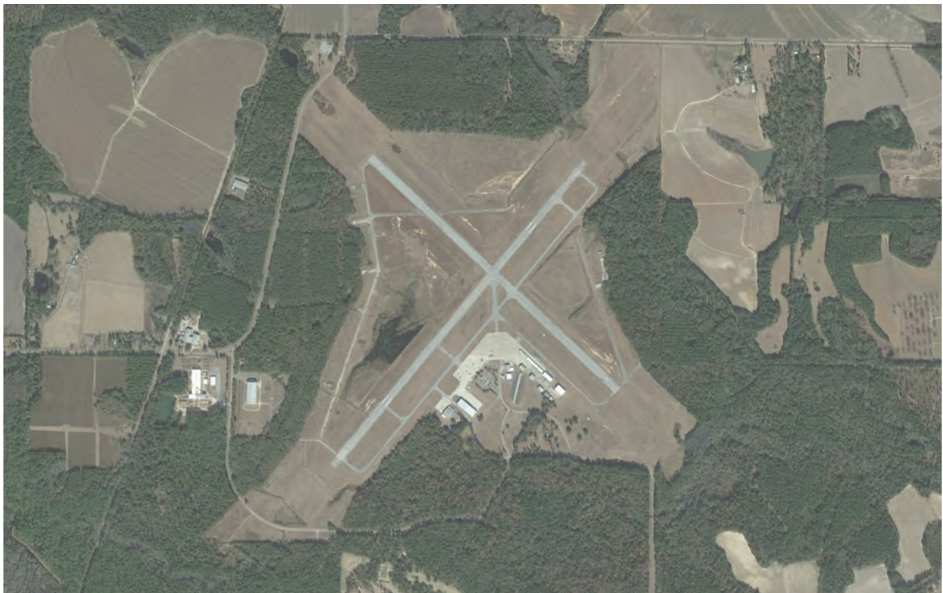
Thomasville Regional Airport
