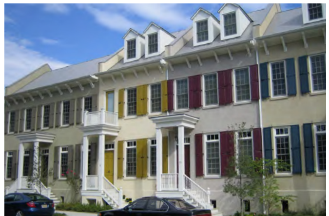
Townhouses with covered stoops, as seen here in Habersham, SC, form a well-defined edge to the street and provide a housing option that currently does not exist in Thomasville.
