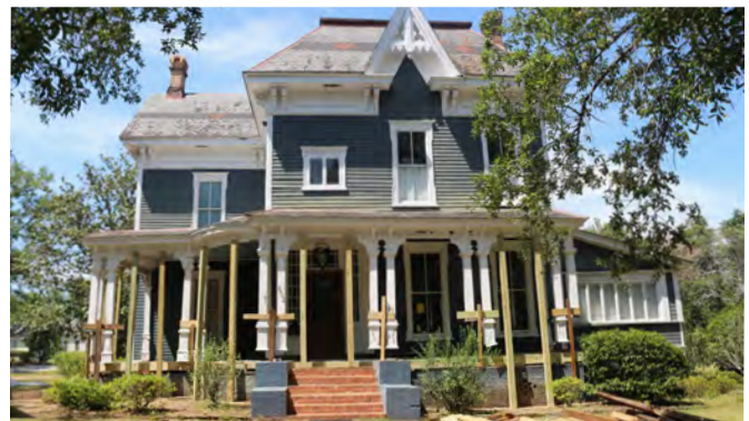
Historic Home Undergoing Restoration
