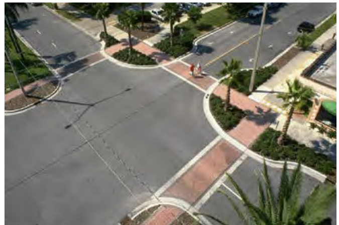
A pedestrian friendly example of curb extensions that can help slow down traffic and reduce crossing distances.
