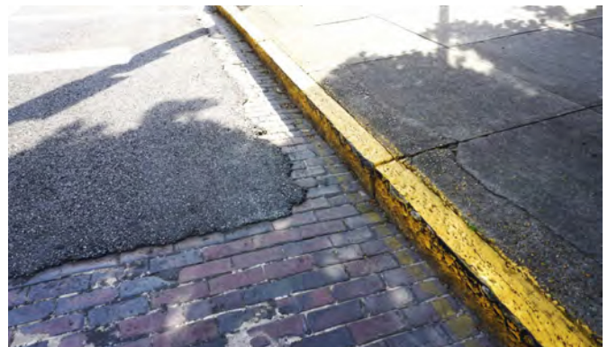
Old meets new - Bricks with granite curbs
